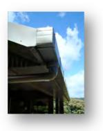
**Wide sloping gutters and downpipes** – these provide for maintenance free gutters, as any leaves big enough to enter the gutter are small enough for the downpipe. The guttering also protects the rough sawn timber fascia from sunlight and the elements. This further reduces the maintenance required in this area of the house.
