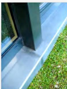
**Stainless Steel Perimeter flashings** – This long lasting innovation provides highly finished detailing and neatly resolves the issue of how the perimeter concrete slab insulation meets the window and wall cladding. The nature of the stainless steel, and the construction of the concrete slab, means that the house ‘floats’ above the ground on a highly insulated pad. There are few, if any, materials in contact with the ground that will be susceptible to deterioration.
