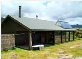
**Orientation** – the house is angled within 15 degrees north for optimal solar orientation. Eaves have been designed to allow sunlight to penetrate in winter whilst providing shading in summer.
