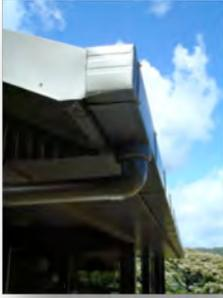
**Wide sloping gutters and downpipes** – these provide for maintenance free gutters, as any leaves big enough to enter the gutter are small enough for the downpipe. The guttering also protects the rough sawn timber fascia from sunlight and the elements. This further reduces the maintenance required in this area of the house.
