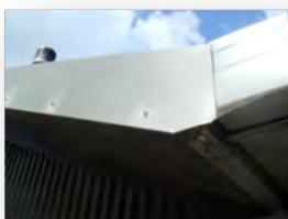
**Bargeboard flashings** – For a minimal extra cost the Colorsteel flashing covers the whole bargeboard – meaning that no additional painting is required for the life of the building. This represents a significant time and paint saving if one considers the job needing to be done every 5-7 years.
