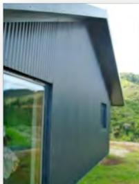
**Use of steel cladding** – the exterior cladding system has a number of advantages from a maintenance and product lifecycle perspective. There is no need to paint the surface as with timber claddings. It only requires a simple wash down once per year with light detergents. The screw fastening system means that individual panels can be removed and sent for recycling if damaged, or at the end of their life, or if a new colour scheme is desired.
