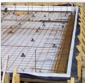
The insulated floor system provides a robust foundation for the house. In the words of the building engineer who worked on Little Greenie the floor is a *“simple, high strength, well insulated raft floor and foundation system which can be used at sites with different ground conditions including those with good ground or cut and filled sites or those with poor ground conditions requiring piles. The reinforced concrete perimeter beam and reinforced concrete ribs within the slab provide a*
